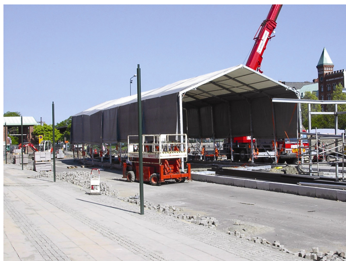
Figure 4.1 Commonly utilised type of weather protecting tent (Jonsereids, 2002).
